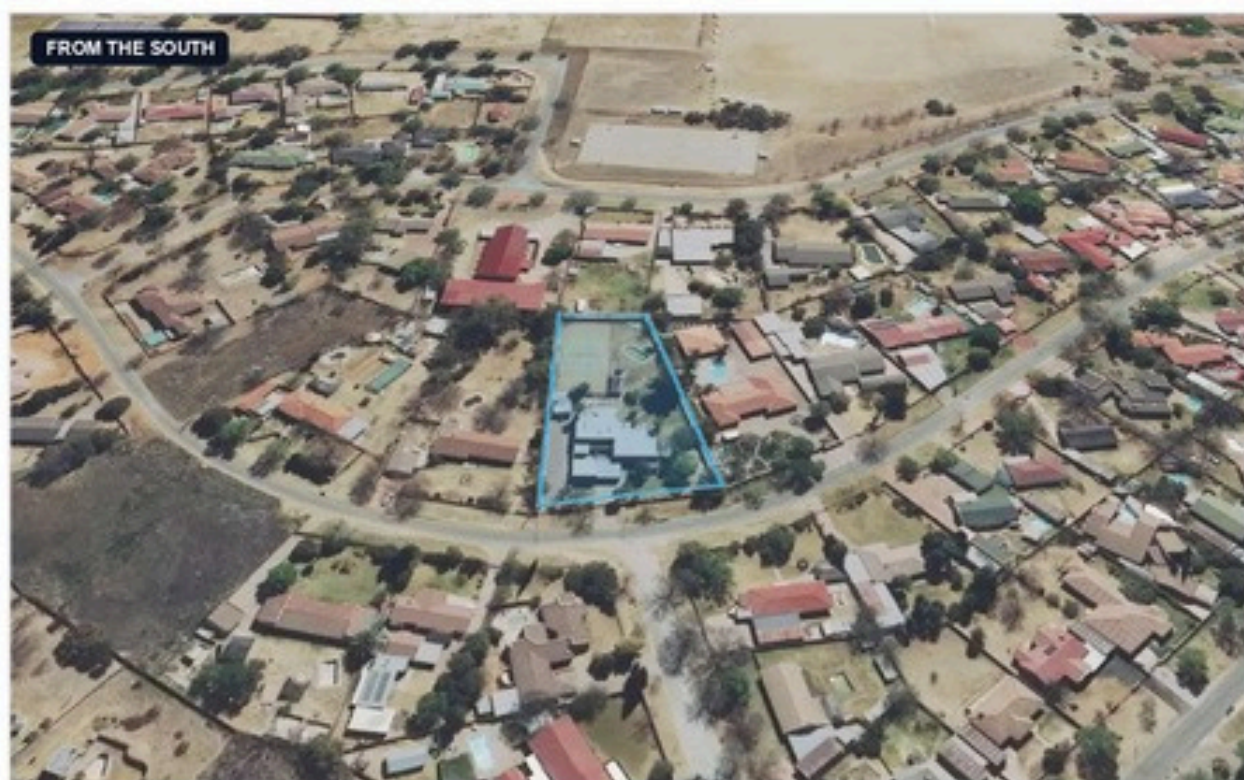
View from the south
