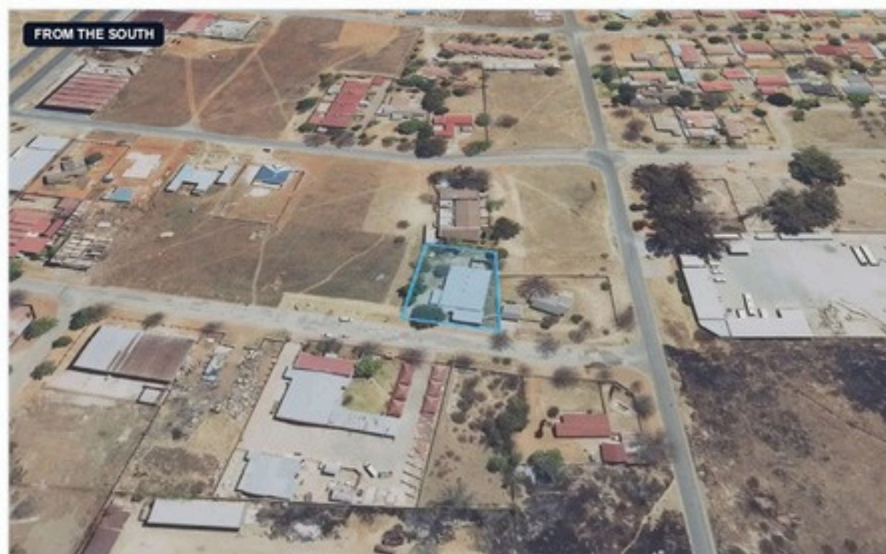
View from the south
