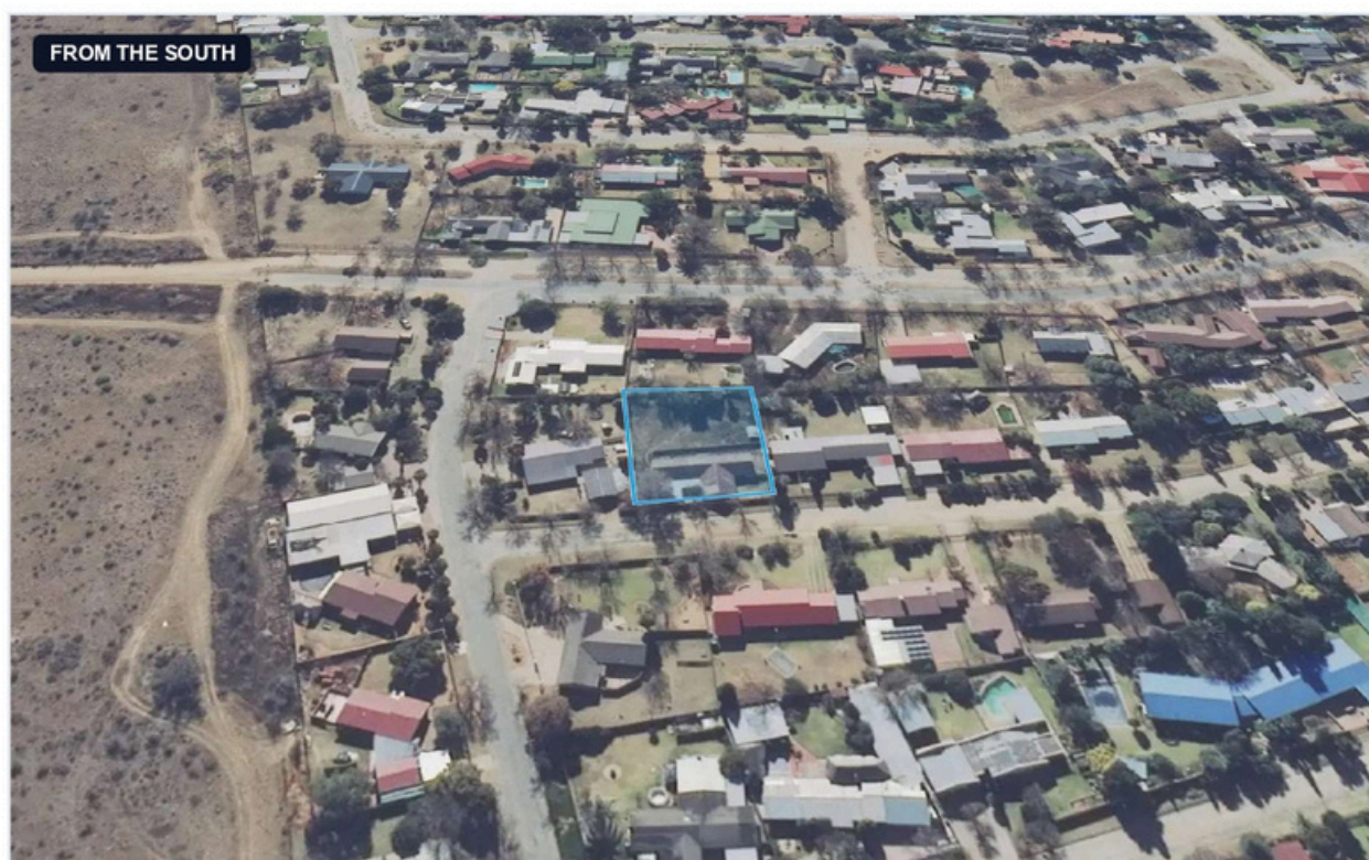
View from the south
